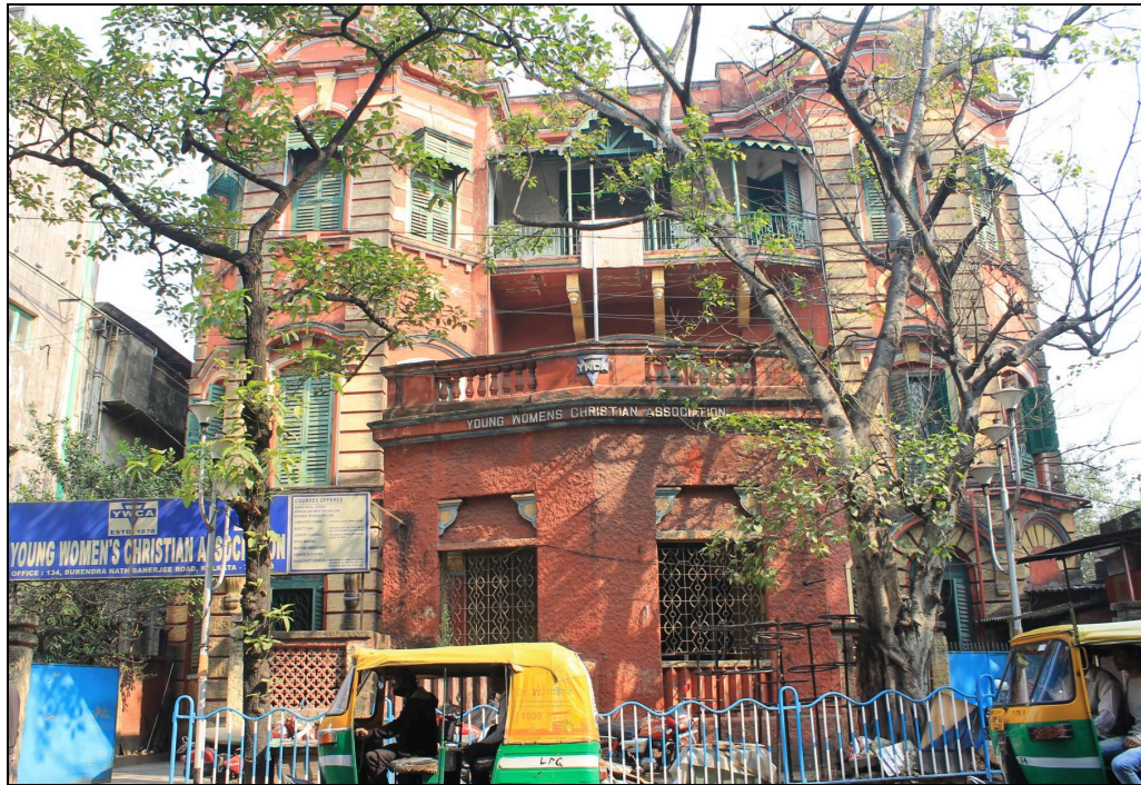
FRONT VIEW OF BURNS HOUSE
